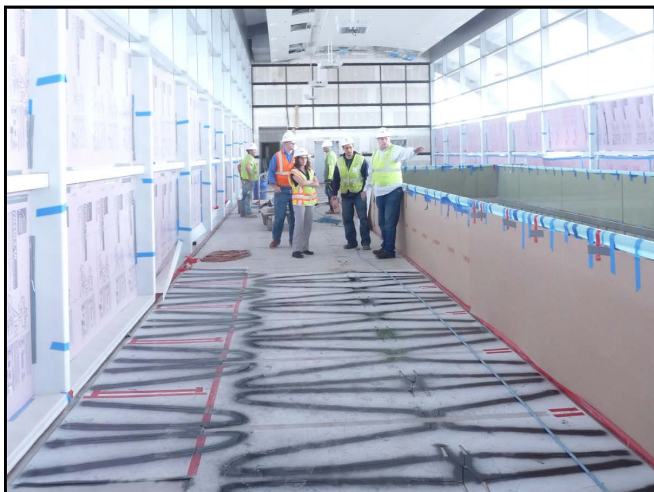
Stencils were used to transfer the design's outline shapes onto the floor.
