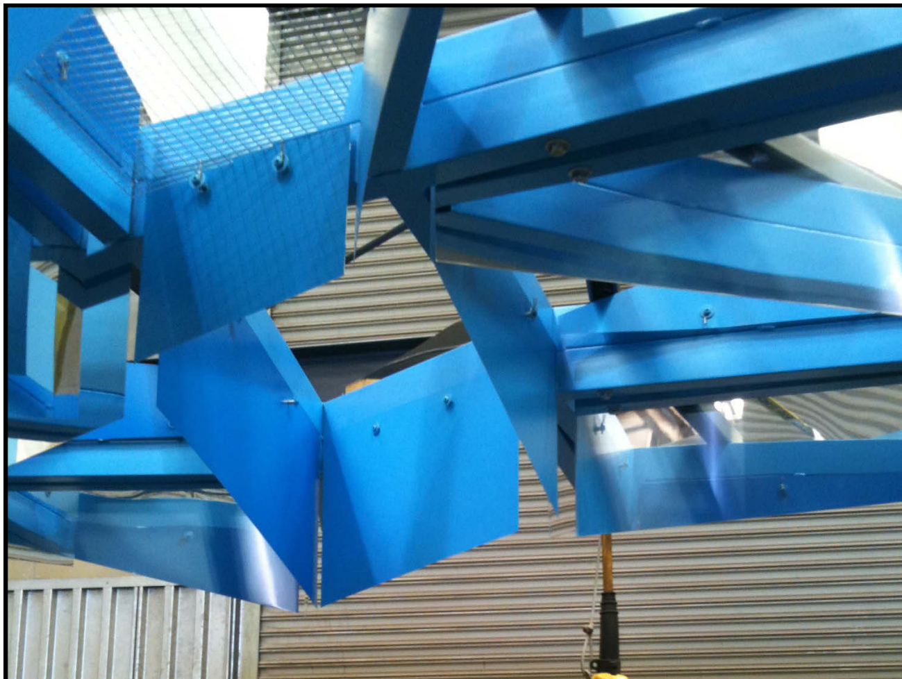
A mock up in CAID Industries shop of a section of the framework with reflector panels attached.
