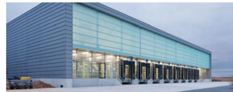
Above: Use a recessed wall plane and glazing to modulate visual impacts of loading bay
